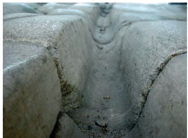
Detail of the impressive furrows –lazy during centuries by the cars– in the stone of the Juyongguan door.
